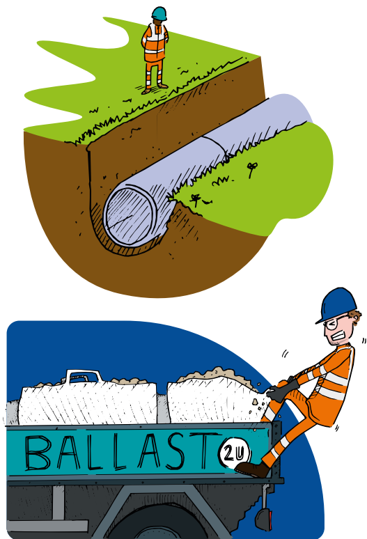
Examples of working at height - control measures must be put in place
